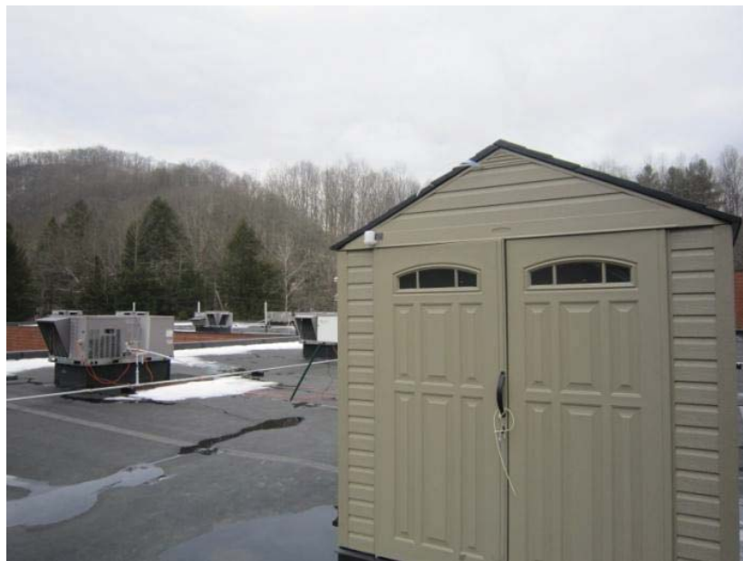
Figure 27. Photograph of equipment shelter at school.
