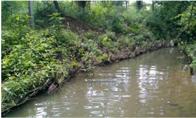
Photo left: Webber streambank stabilization project. Area was graded to a less steep bank angle and protected with brush mattress, live fascines, and live stakes. No excavation was done due to limited access, and impacts by mobilization were avoided.
